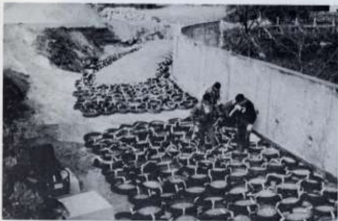
Reduce active earth pressure at Mende (Lozère)
