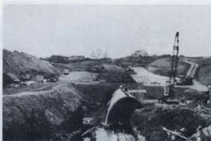
Creation of arching at Monistrol-sur-Loire (Haute Loire)
