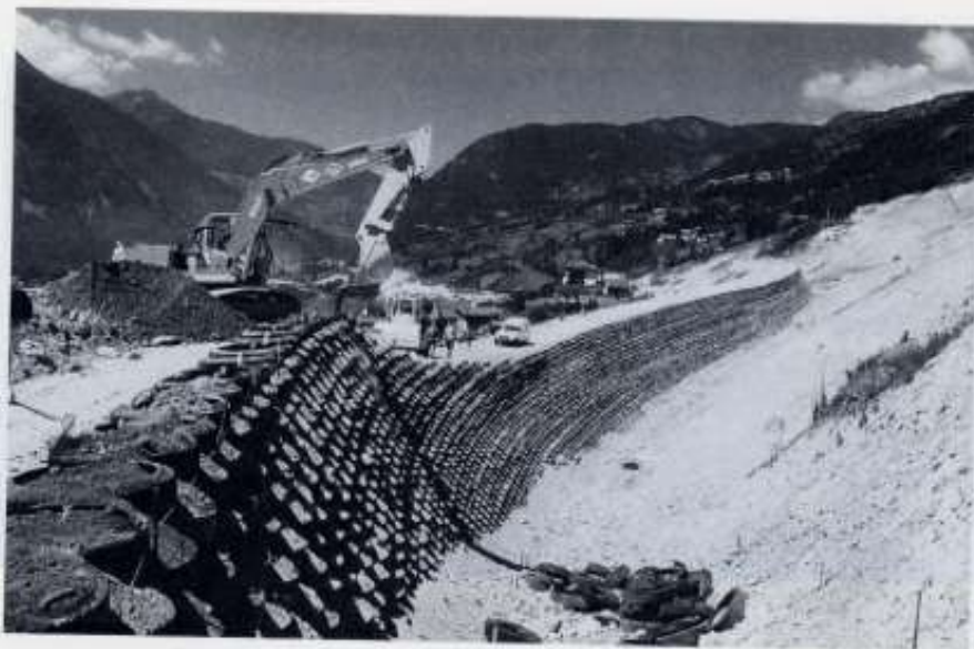
Energy absorption at Vallabonnette in existing drive with rockfall
