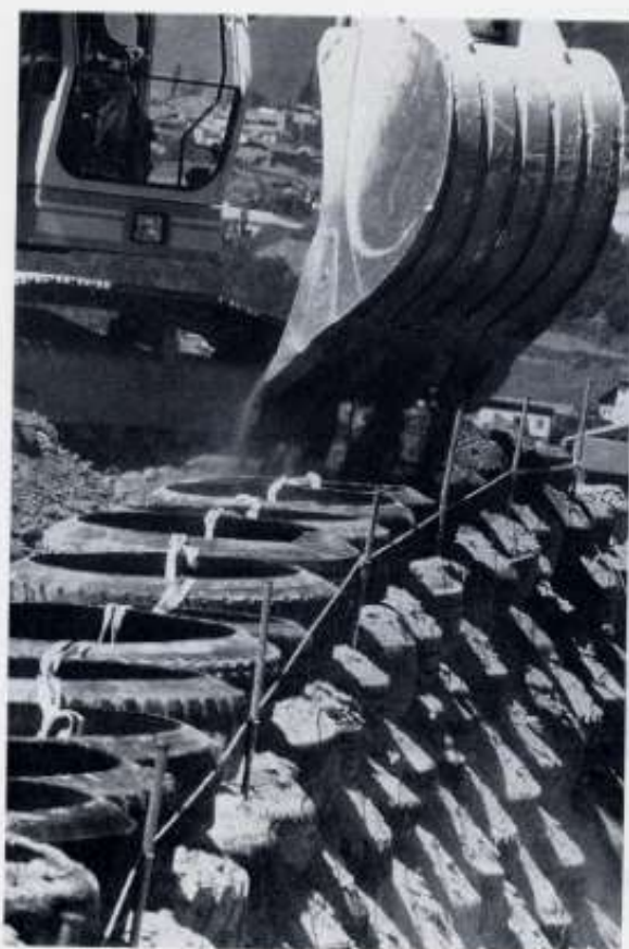
Energy absorption at Vallabonnette in existing drive with rockfall
